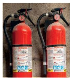
A fire extinguisher or two, of the proper type and current charge, is a low cost, very worthwhile addition to any area with wood, wood dust, and chemicals
